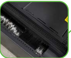
Brush cable managers in floor of cabinet
