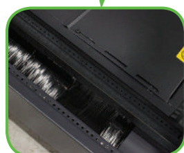
Brush cable managers in floor of cabinet
