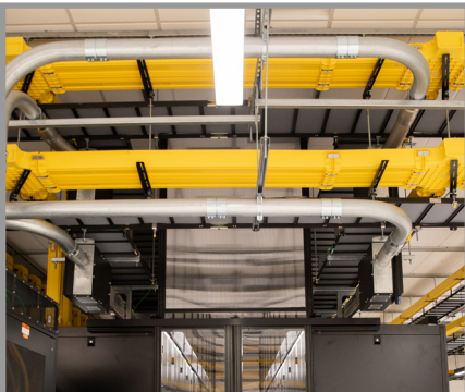
Cable Runway Systems
